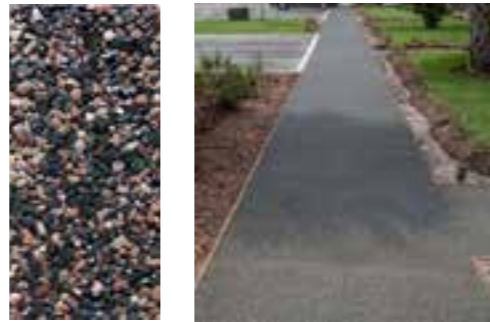
Flexi-pave recycled bound surface - recycled rubber and aggregate surfacing
