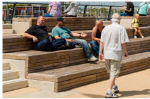
Untreated timber seating steps
