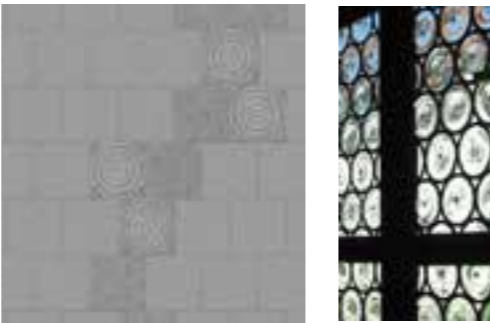
Natural stone setts and small flags with textured surface referencing the crown blown glass produced on site
