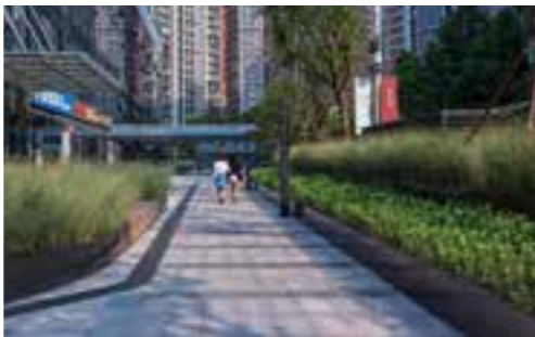
Steel edging, predominately laid flush with 150-450mm raised edge on the podium
